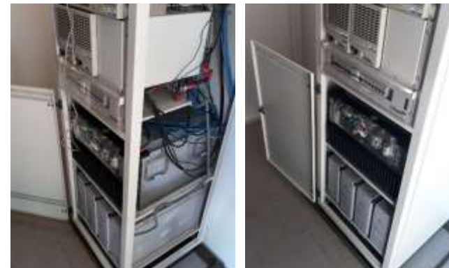
LABEL-FREE 48TL200 (suitable with 23" cabinets) It's a 48V 200Ah battery block (9,6kWh)
