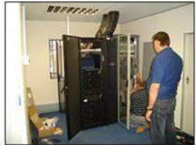
Installation of iSX solution Vryburg
